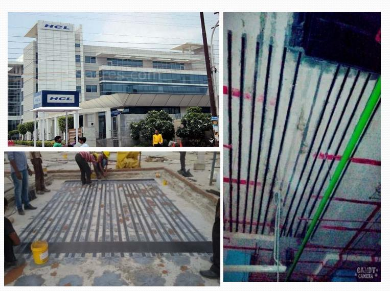
Slab Strengthening work with Retrofitting, Carbon Laminate And Carbon Wrapping.
