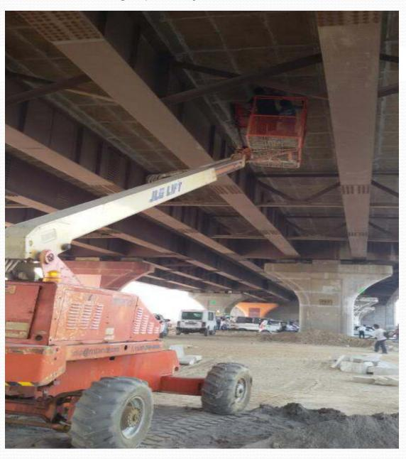
BRIDGE RETROFITTING WORK WITH EPOXY GROUTING & CARBON LAMINATE, WRAPING
